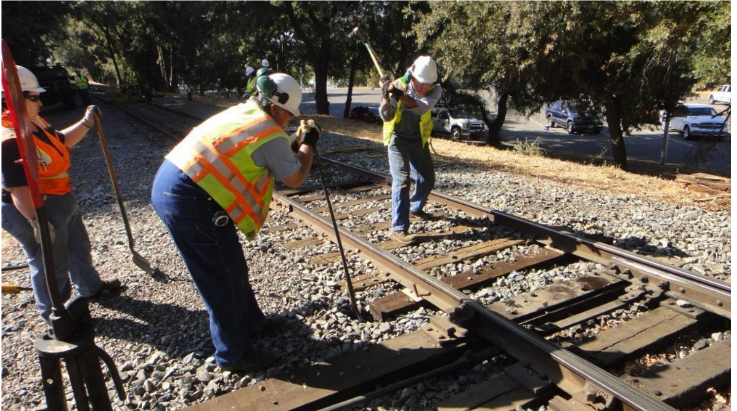
Steve demonstrating his world famous “windmill” spiking technique with the spike maul. He never misses.
