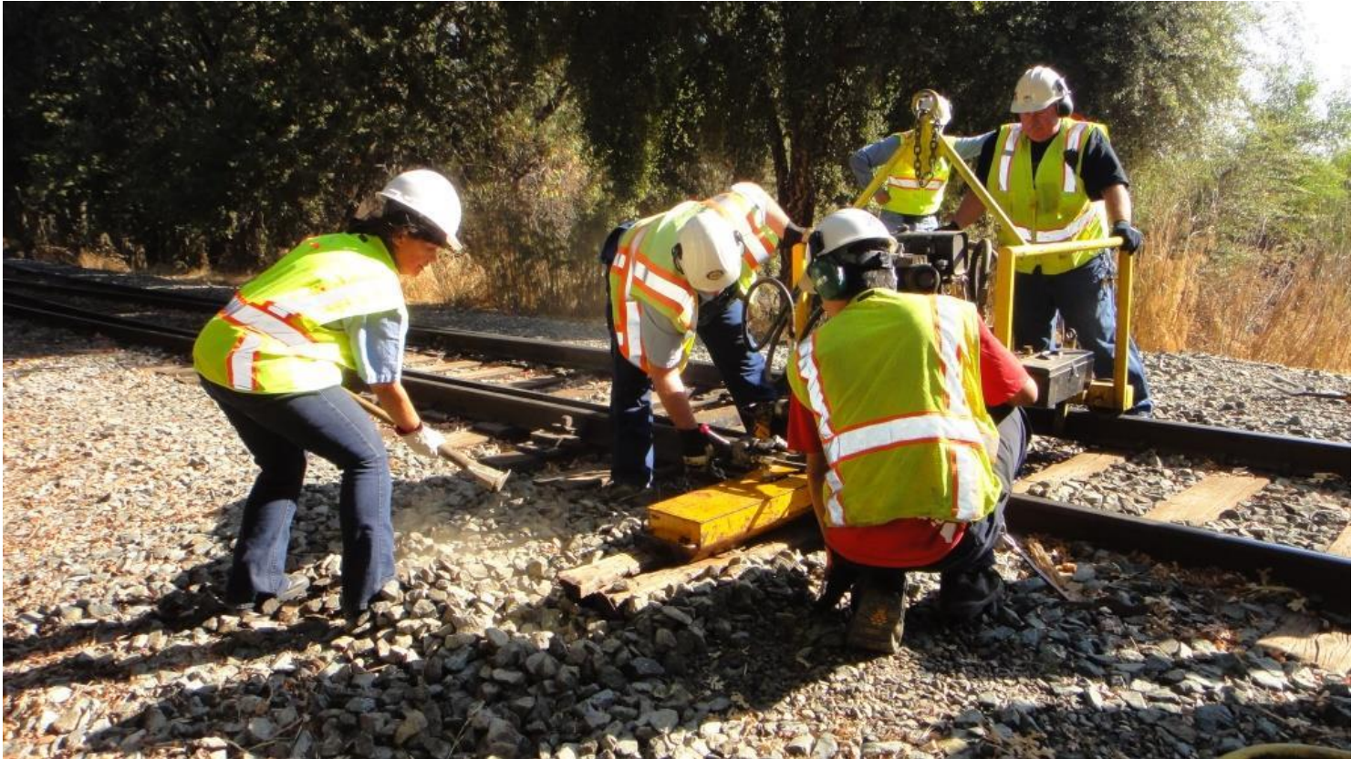
Pam digs out the end of the tie to help it move more freely as Chris, Harry, and Josh engage the chains on the section-gang machine in an attempt to prevent crushing it.
